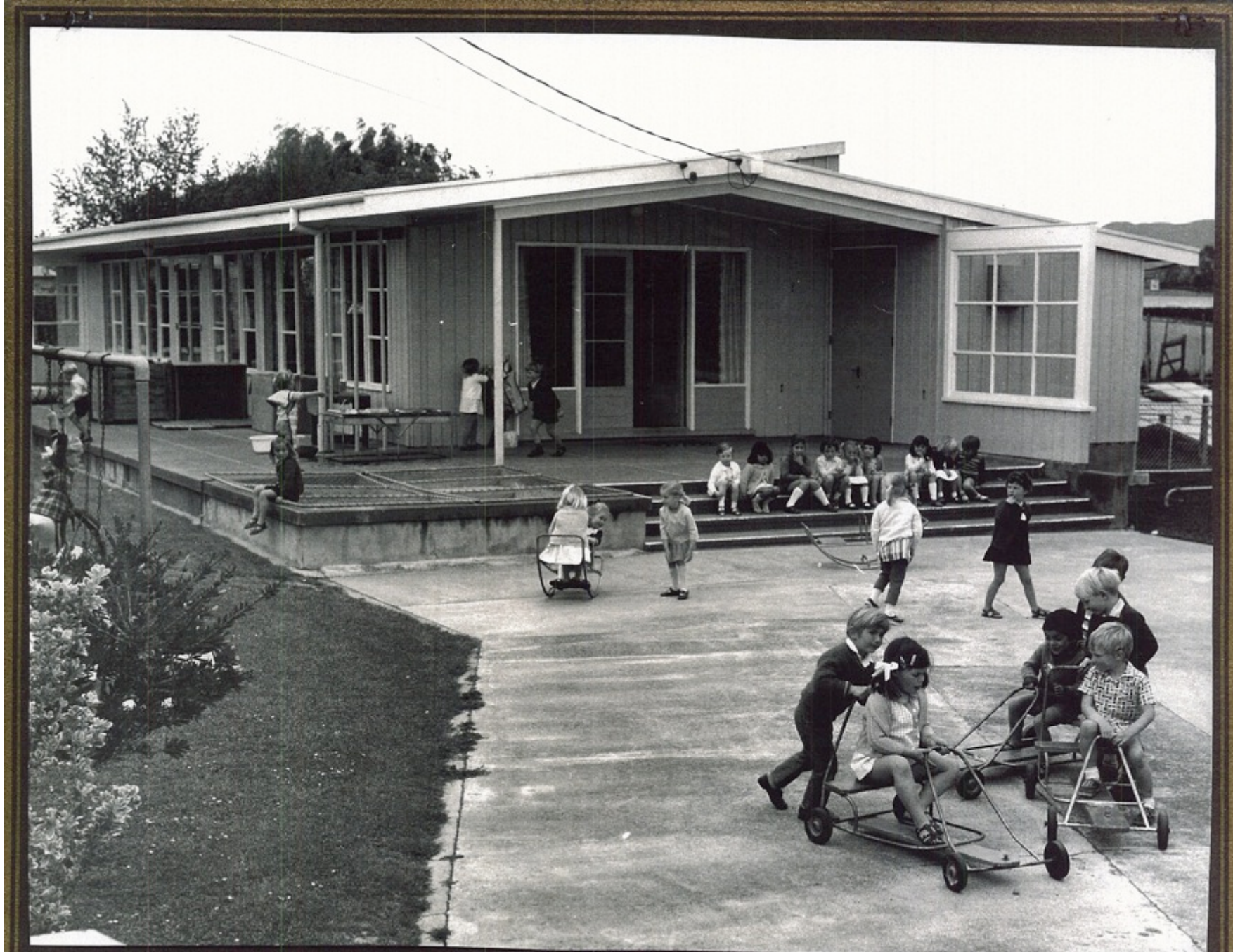
Parkvale Kindergarten, Hastings
